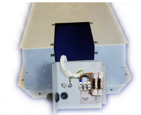
Fig.1.0 Heater with terminal cover open
